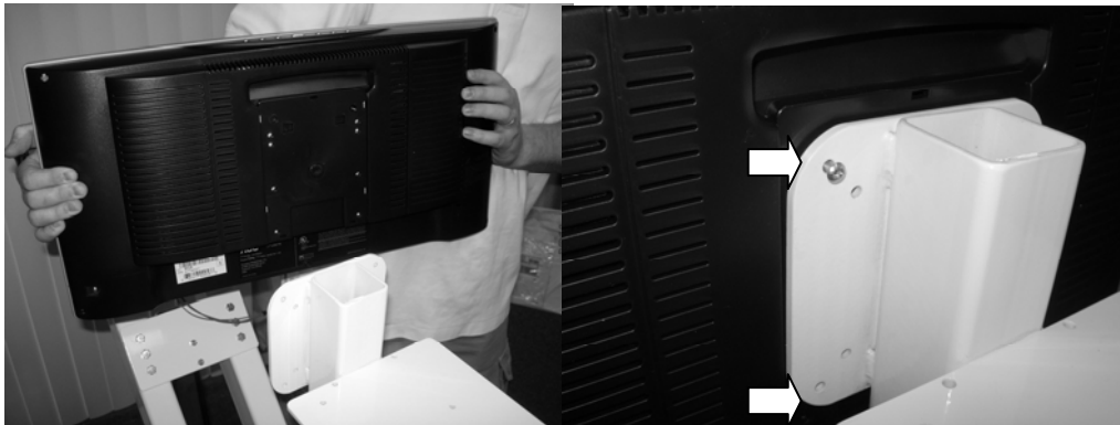
Figure 3.1: Mounting the LCD TV to the GameCycle.
